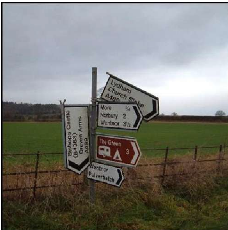
Damaged signs on Strategic Route; Target Response Time Cat 3.
