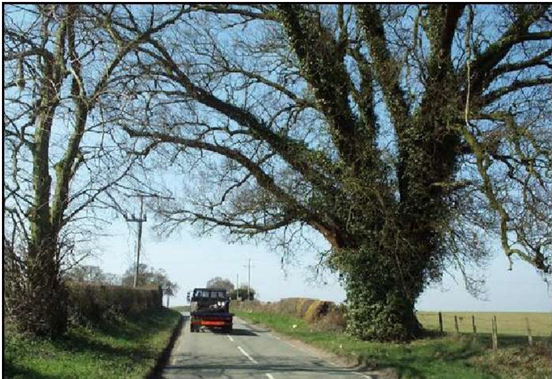
Overhanging tree, see note 3.
