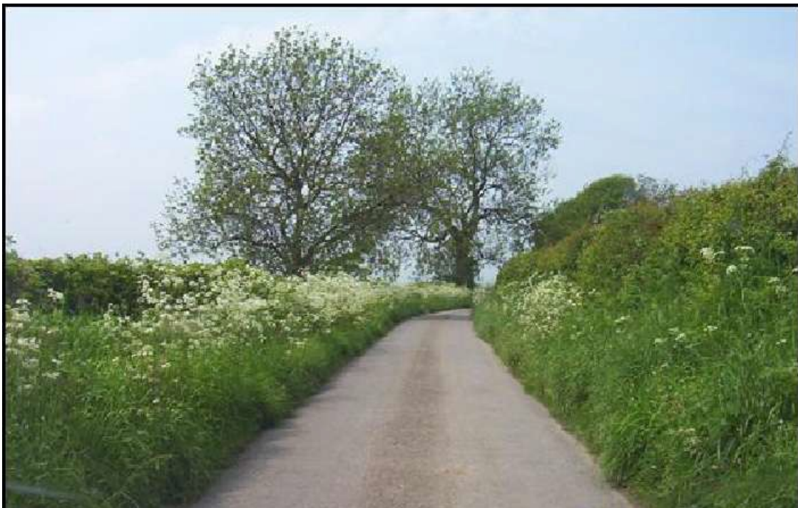
Local rural road overgrown by vegetation restricting visibility: Target Response Time Cat 2.
