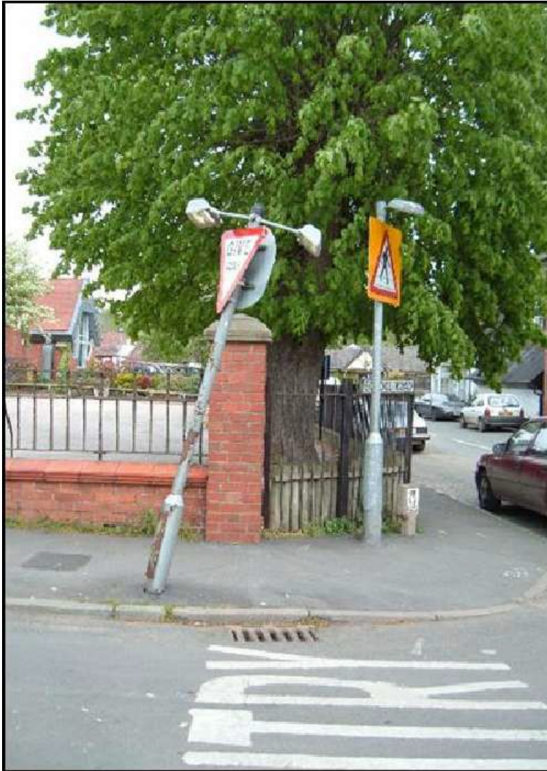
Leaning sign Local urban: Target Response Time Cat 1.
