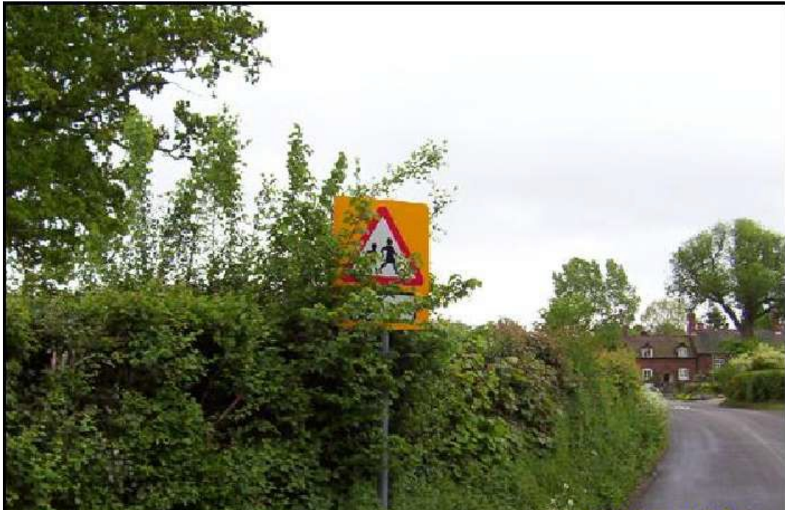
Regulatory sign obscured Link Road: Target Response Time Cat 1.
